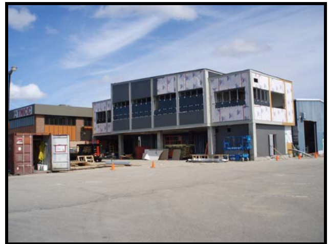
Office extension in progress
