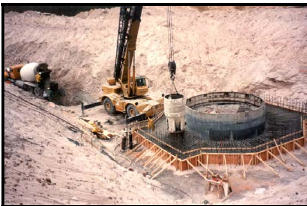
Shaft collar construction
